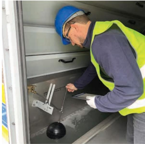
Figure 24: Mechanical water level control
