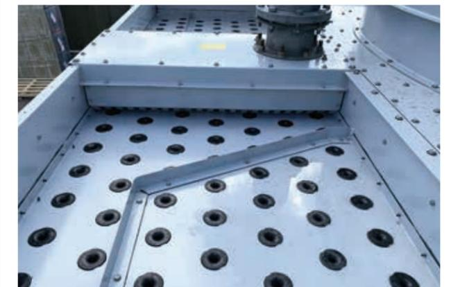
Figure 23: Hot water basin with gravity water distribution
