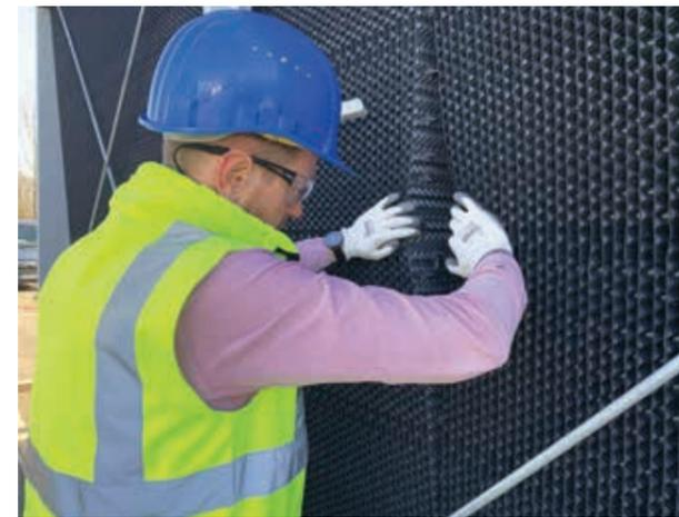
Figure 28: Heat transfer surface
