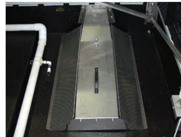
Figure 21: Cold water basin strainer
