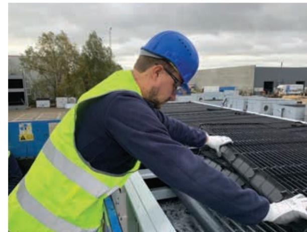
Figure 29: Drift eliminators
