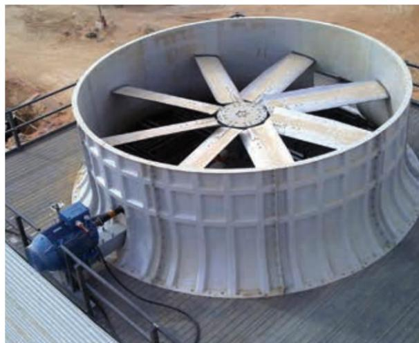
Figure 32: Mechanical drive system
