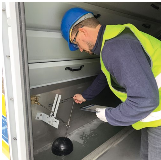
Figure 24: Mechanical water level control
