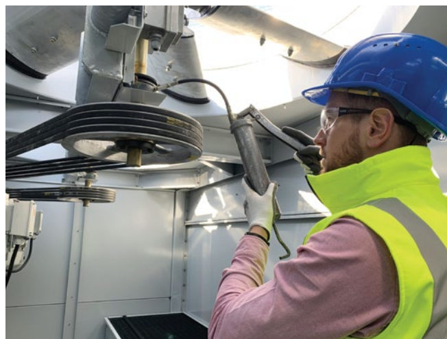
Figure 27: Greasing the bearing
