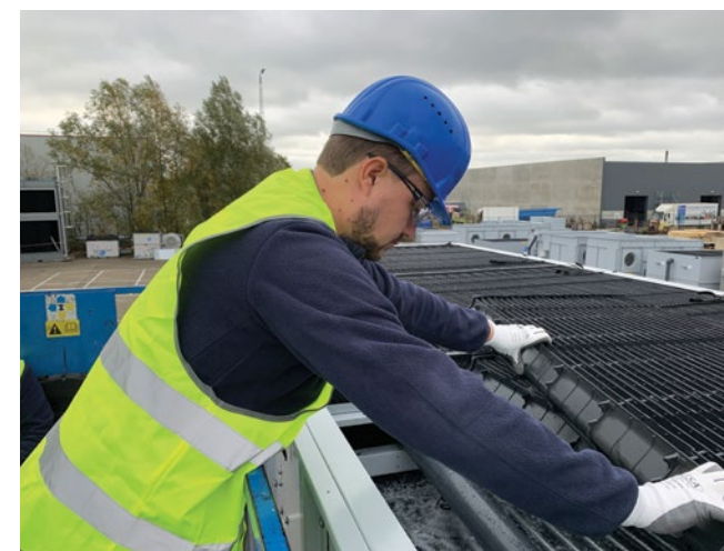
Figure 29: Drift eliminators
