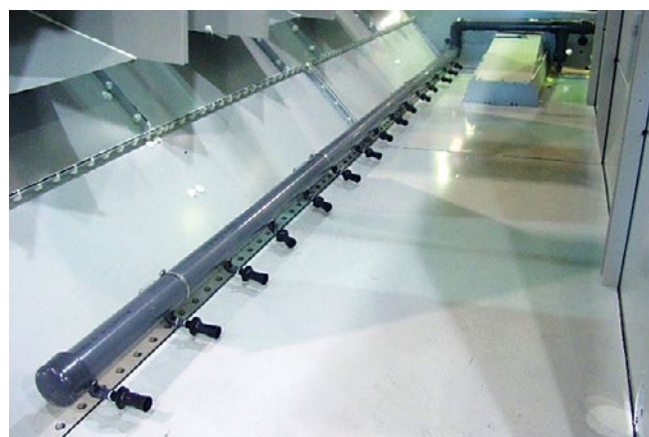
Figure 31: Basin sweeping piping
